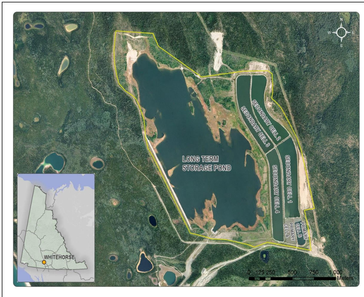
Figure 1. Location of the Livingstone Trail Environmental Control Facility, Yukon, Canada, as well as configuration and naming of the seven treatment cells.
