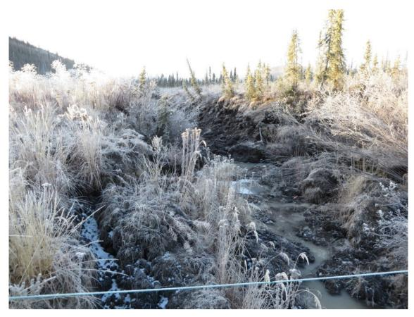
Figure 4.6.11. Thermal erosion in the ditch, facing southwest.
